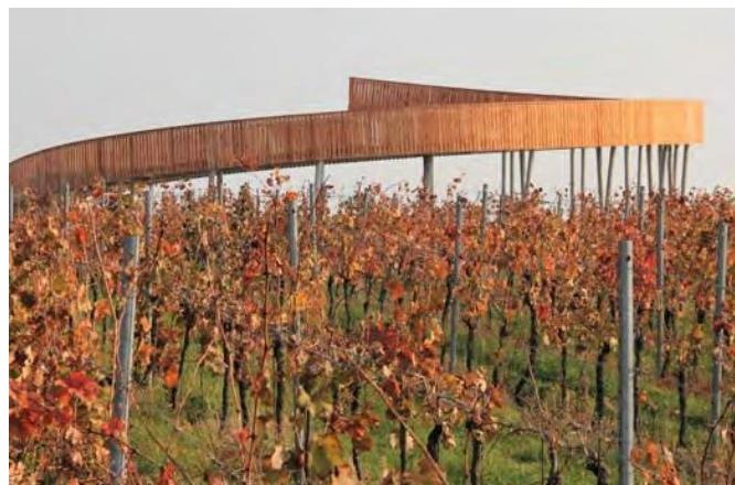
The walk above the vineyards, Keeog desing, Netfloor USA
